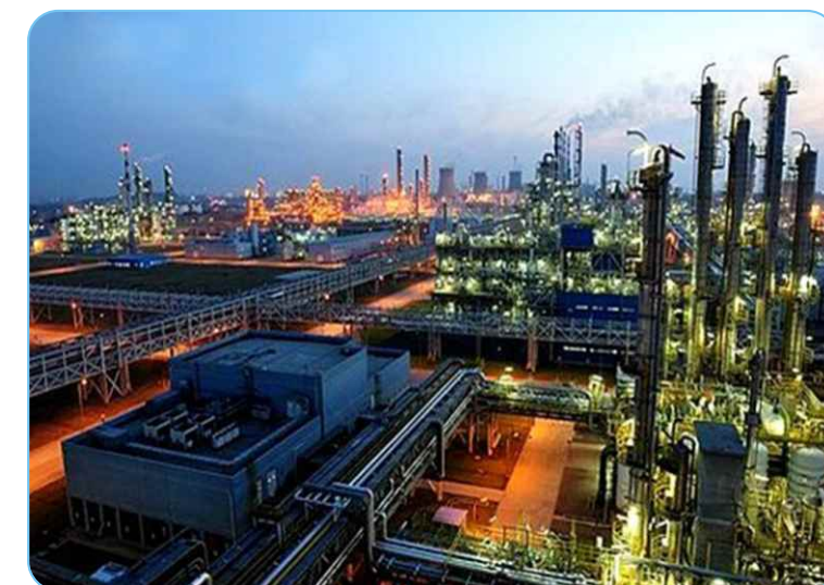
化工厂一角 Part of the power plant
