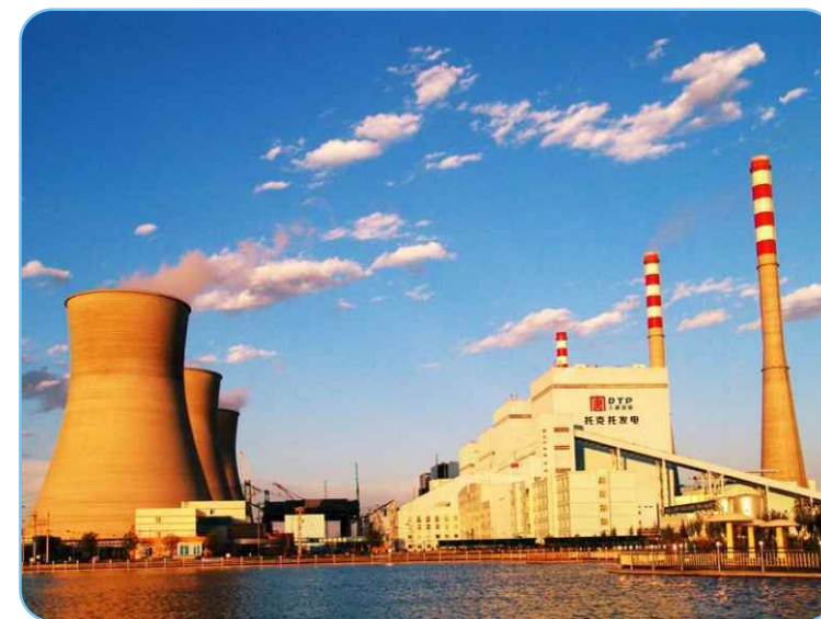
化工厂一角 Part of the power plant
