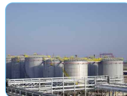
储罐 Storage tank
