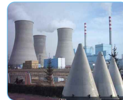
煤斗及烟筒内衬 Coal bucket and pipe lining
